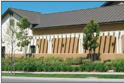
3.2.1.7 b) Low rise, landscaped screening walls contribute to a more attractive environment.
