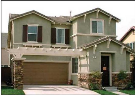
3.3.6.11 a) Recessed garages give importance to the entry and create a pedestrian friendly neighborhood.
